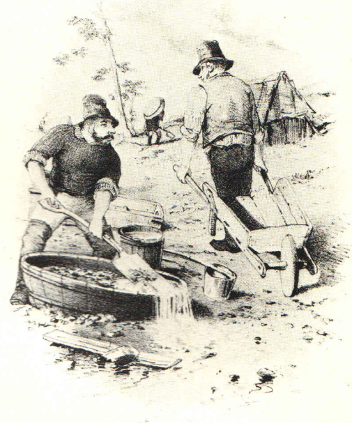
Many diggers preferred to wash the soil in a cask before using the cradle to extract gold.
